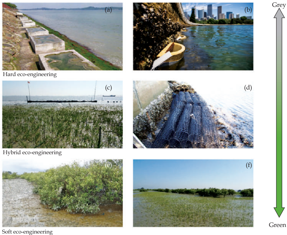
Fig. 1.1 Different ecological engineering approaches incorporated into coastal defences: (a) Traditional embankment with concrete tide pole to enhance biodiversity (Singapore); (b) Sea wall with water retaining feature to enhance biodiversity (Sydney); (c) oyster breakwater reefs to enhance marsh vegetation (Bangladesh); (d) Artificial substrates used in front of sea wall for oyster reef formation (Florida); (e) planted mangrove forest (Bangladesh); and (f) Natural salt marsh facilitated by planted mangroves (Bangladesh). [Photographs: a, b, d were taken from different internet sources].
