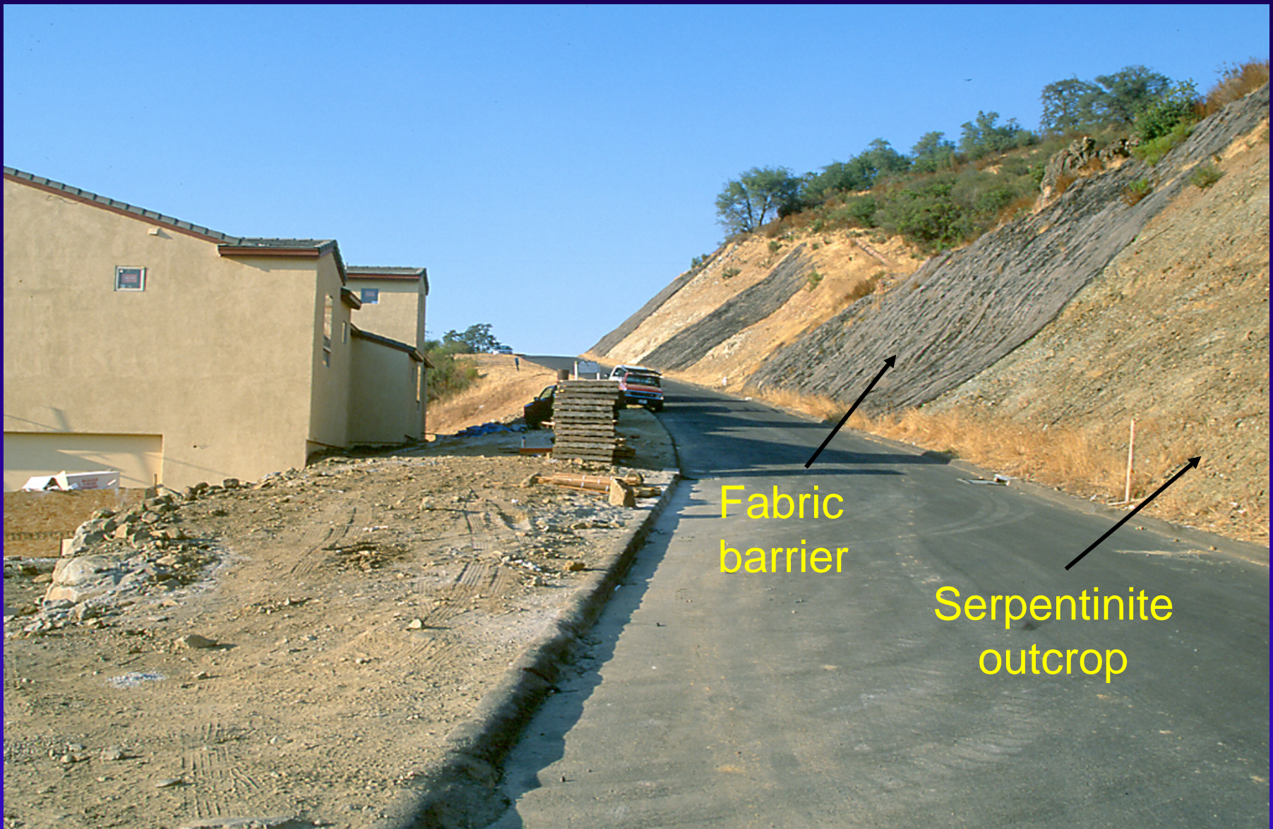
New homes being constructed on the side of a hill cut into serpentine-bearing rock.
