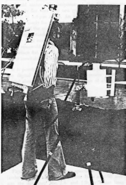
**Fig. E-1. Portable field reflectance spectrometer in operating position. Backpack contains the amplifiers, power supply, and digital recording electronics. Optical head contains the chopper, circular variable filter, thermoelectrically cooled detectors, and preamplifiers**
