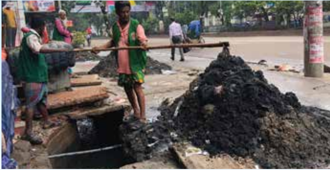
Manual Drain Cleaning
