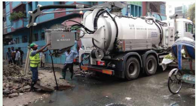
Jet & Sucker Clearing the Drain Blocks
