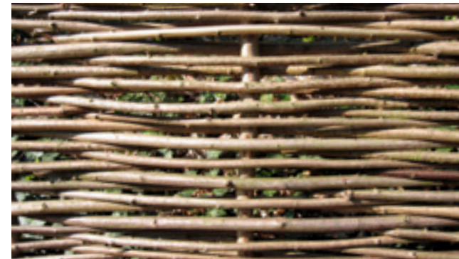
Figure 6.2: Detail of a willow branch wicker
