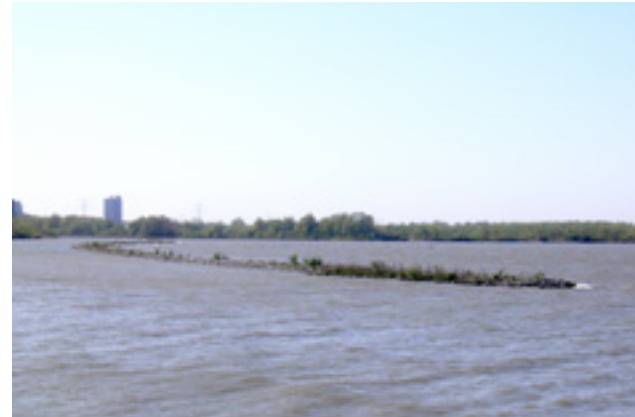
Figure 5.2: Breakwater at the coast near Muiden
