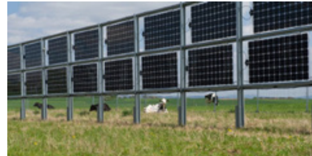
Figure 5.10: East-west facing vertical bifacial PV array along agricultural use
