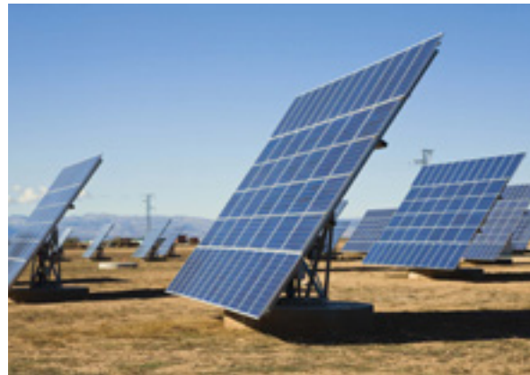
Figure 5.14: Example of a dual axis solar tracker
