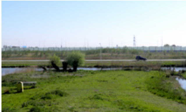
Figure 4.8: Converging large infrastructures along an old polder
