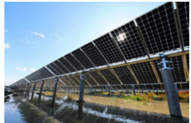
Figure 5.9: Fixed bifacial PV array above surface water in the US
