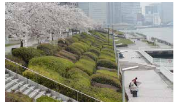
The Super Levee concept was first tested (with success) in Tokyo Japan. The elevated cityscape integrated with existing buildings and provided a richly textured public environment.
