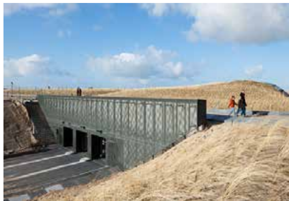
Katwijk coastline in the Netherlands provides transportation, recreational, ecological, and resiliency services to its community.
