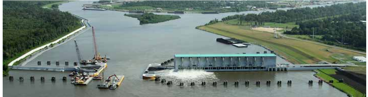
The Gulf Intracoastal Waterway West Closure Complex includes pumping mechanisms to maintain river flow during high water.
