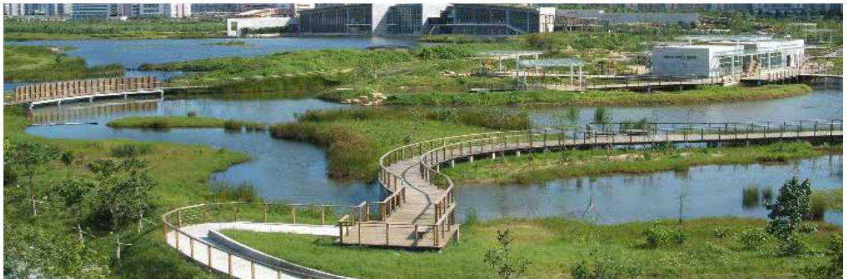
Stormwater treatment wetlands slow down runoff, clean the water, and provide wave and storm surge buffers during over-topping events and king tides. Equally important is their value as habitat matrix to threatened Bay Area shorebirds.
