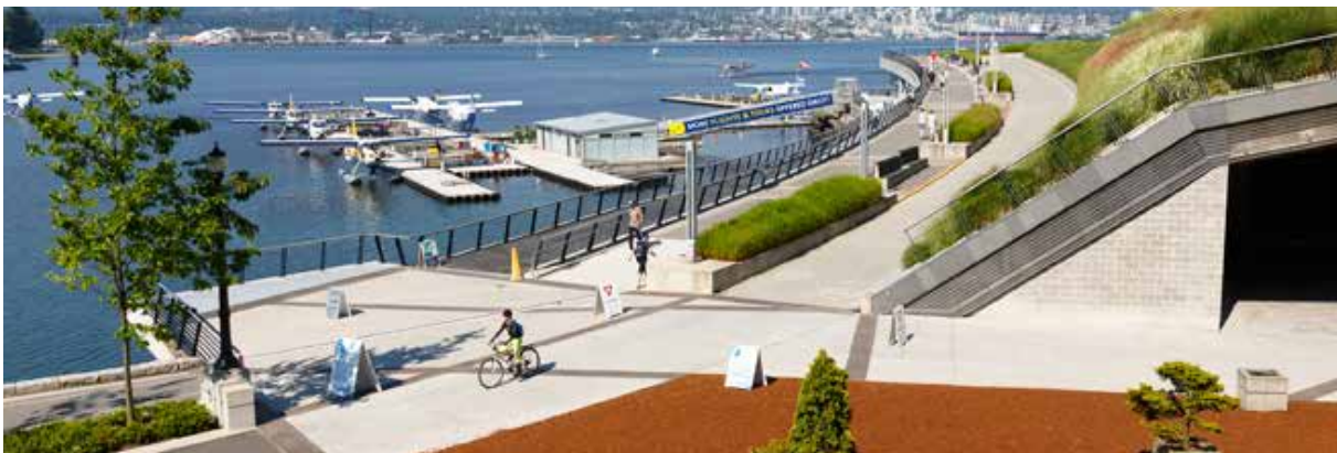
Traditional levees can be positioned as game-changing social infrastructure that reinvests in our waterfronts.
