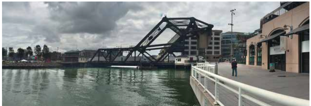
The 3rd Street bridge and promenade outside the ballpark present unique challenges in maintaining asset value while protecting them.
