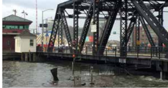
3rd Street Bridge during a high “King Tide”
