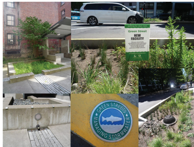
Figure 10. Some green infrastructure examples in the City of Portland: stormwater planters (left) and green streets (right)
