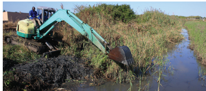
Figure 34. Maintenance of the channel by a digging machine
