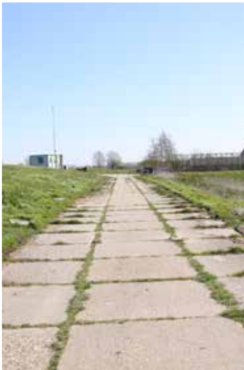
Figure 8.4.5.5: Stelcon plates on site
