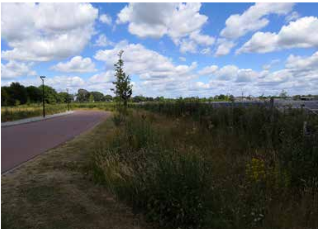
Figure A.2.10: View from local road towards PV system
