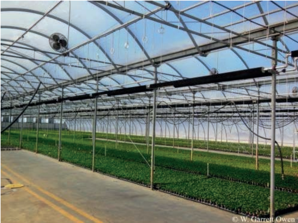
Figure 25 Multi-span greenhouse with a "snow" pipe below the gutters.
