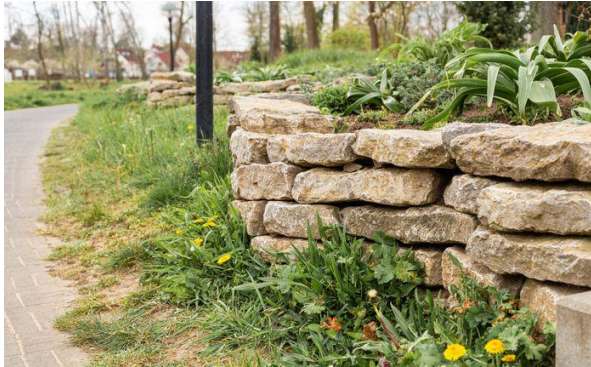
Figure 28. Example of a stapelmuur: a loosely stacked wall that provides a lot of opportunities for biodiversity. Source: ff25 shutterstock, n.d.
