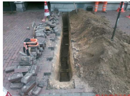
Figure 21 - Test slot in de Kamp showing underground infrastructure.
