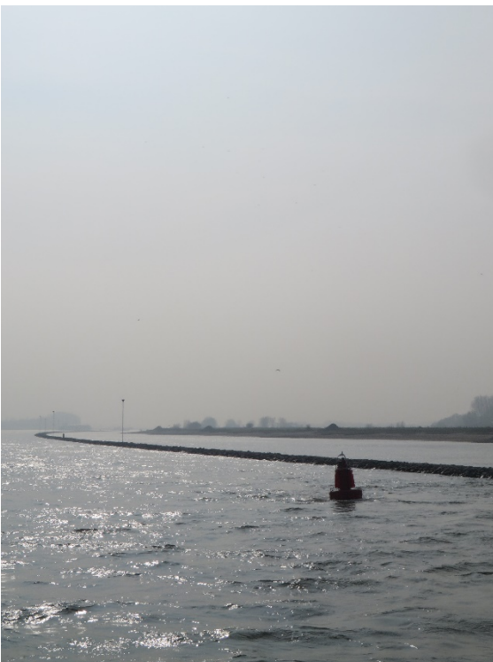
Figure 2: A longitudinal training dam seen from the fairway, where the buoy indicates the foot of the slope.
