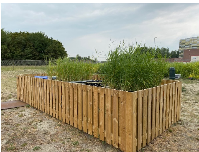
Figure 3: Constructed wetland pilot in Terneuzen, the Netherlands, effectively removing conditioning chemicals from cooling tower wastewater.
