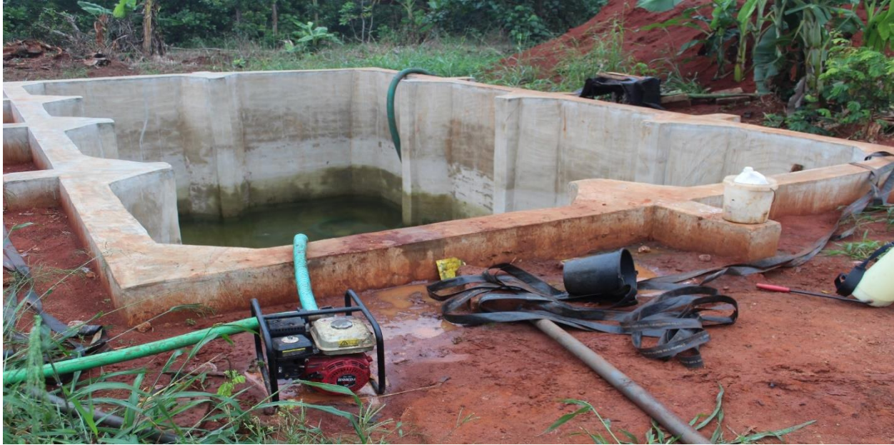
Figure 11: Concrete storage tank for underground water storage for irrigation
