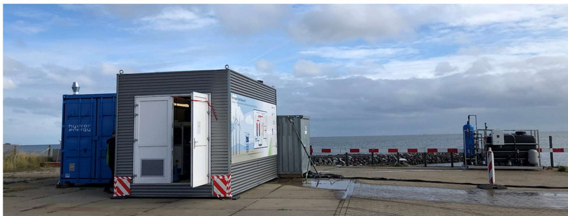
Figure 8: PEMWE (blue container) and MD (grey container) installation with the installed seawater intake at the right head of the dock.
