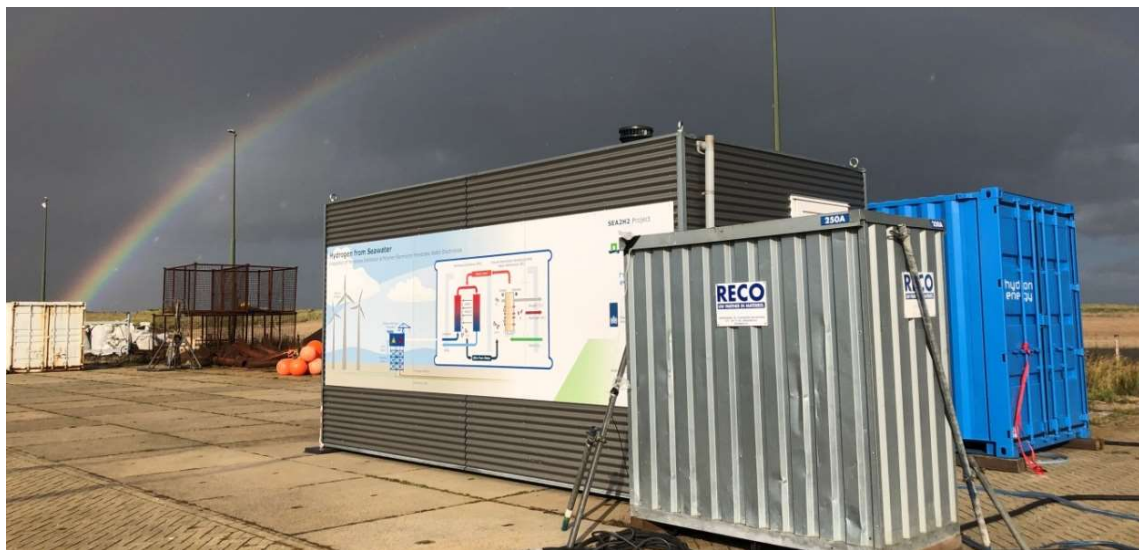
Figure 7: Visual on the MD container, the power distribution box (grey RECO container) and in the background the blue container with the PEMWE installation
