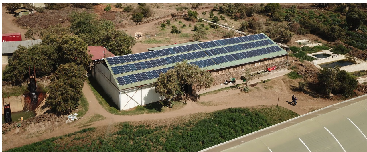
Solar panels on a rose farm in Kenya (Photo: Sebastian Noethlichs)
