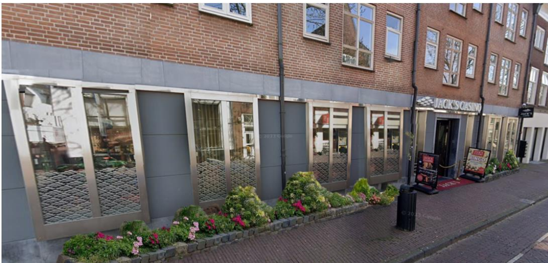
Figure 26 After adding a green façade to Jack's Casino
