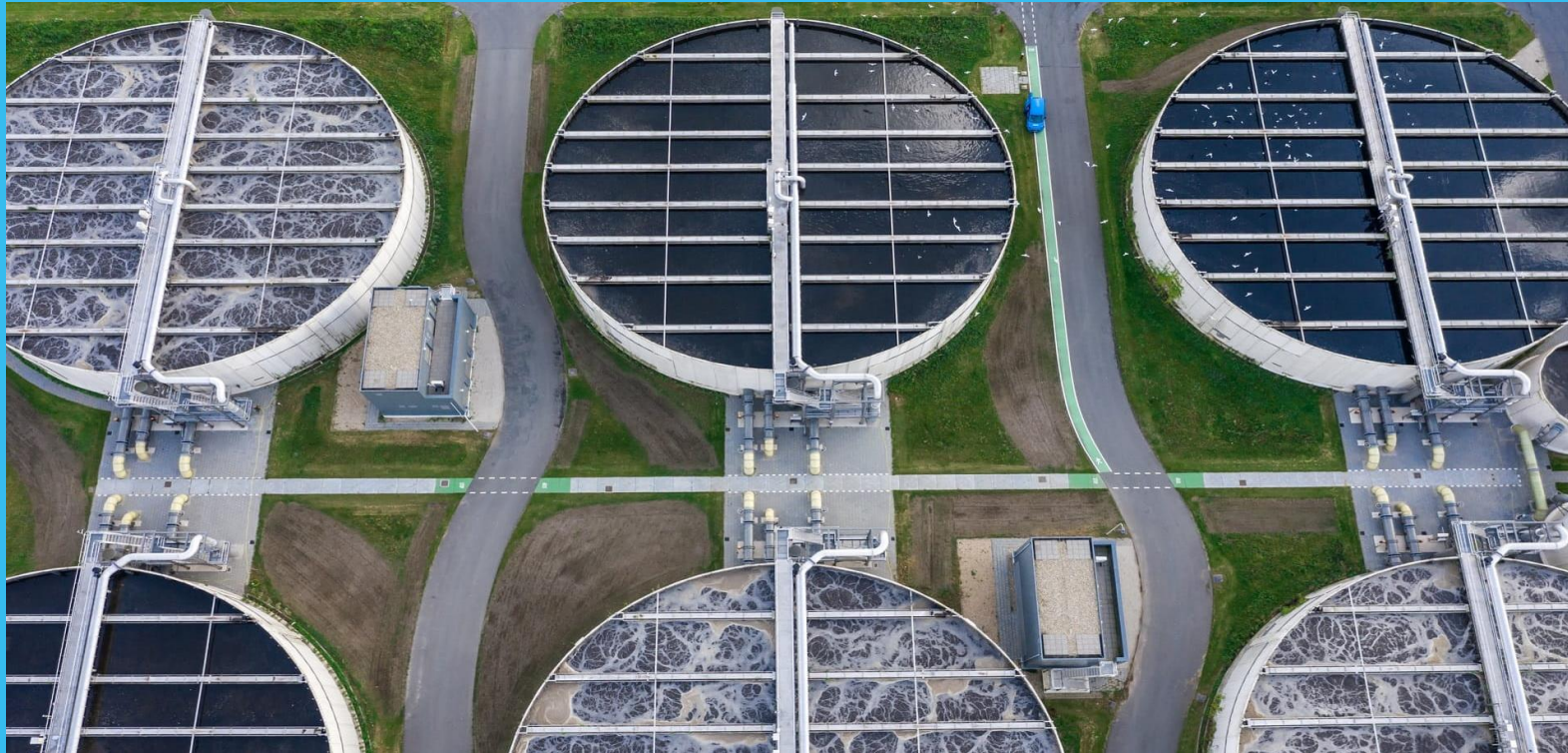
Nereda wastewater treatment plant Utrecht, Netherlands
